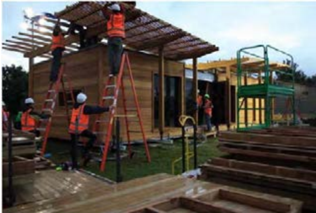
Figure 5 (on the left). Roof panels being assembled on site, 2011. (image: First Light Studs. Photo credit: Ron Blunt).
