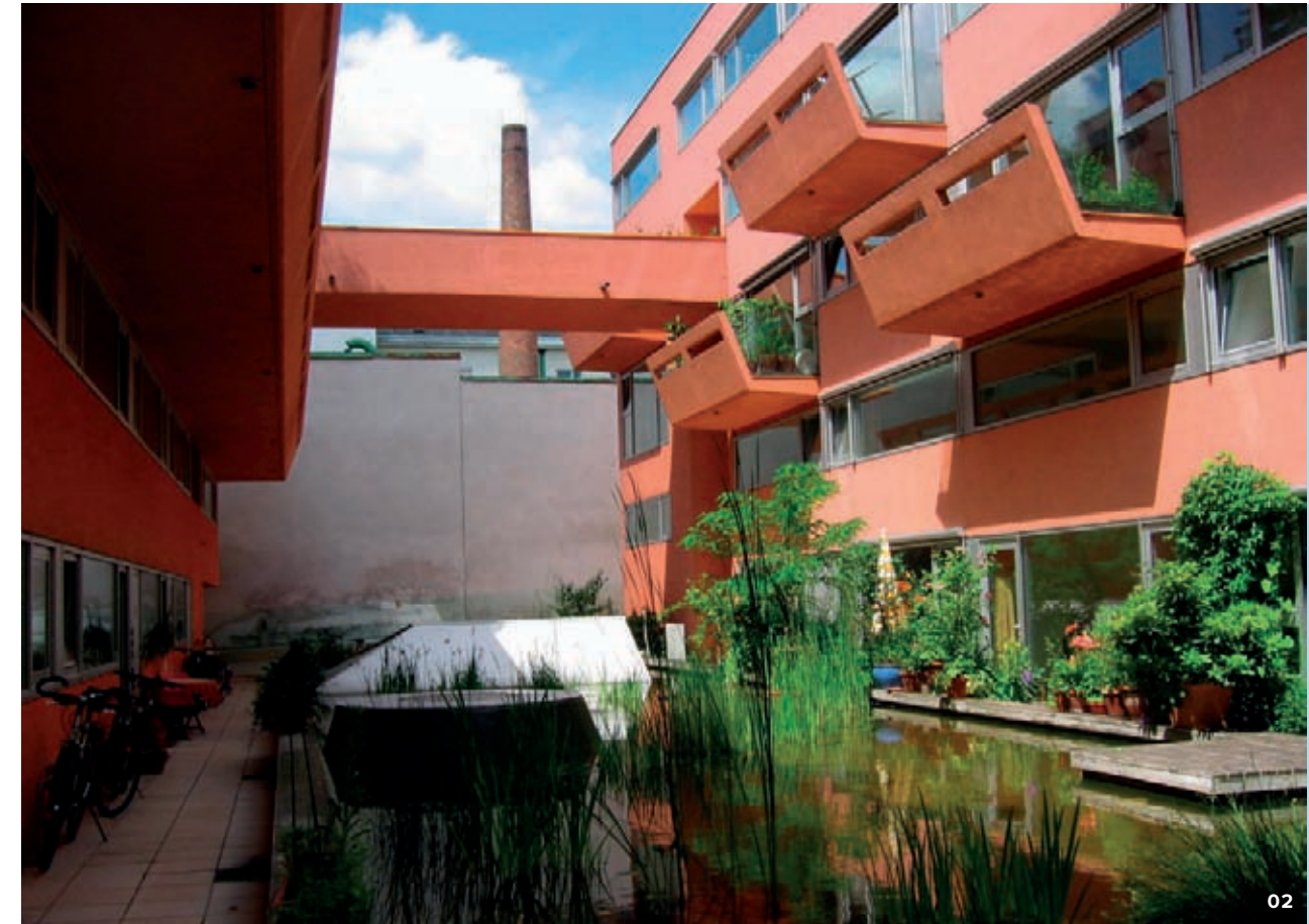
02 The Sargfabrik in Vienna, by BKK Architects 2, is Austria’s largest self-governing housing and cultural project. It was created by a group of people who were discontent over the expensive housing market and wanted a project designed for families.
