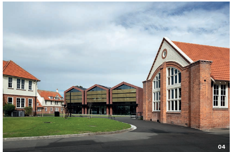
04 The new Administration Building, seen here with the museum and Big School on the left and the library on the right.
